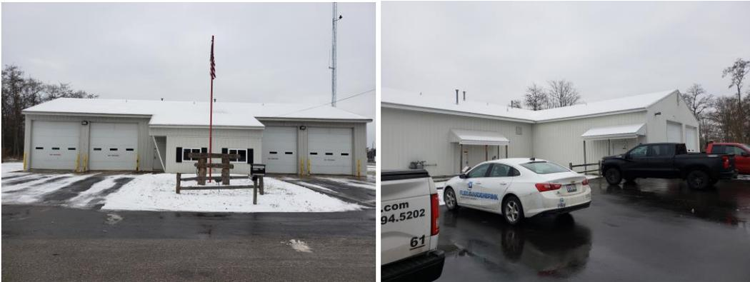
The existing building is wood post-frame (pole barn) construction. The truss-bearing (ceiling) height is approximately 13'-3", allowing 12' high garage doors having low headroom tracks.
